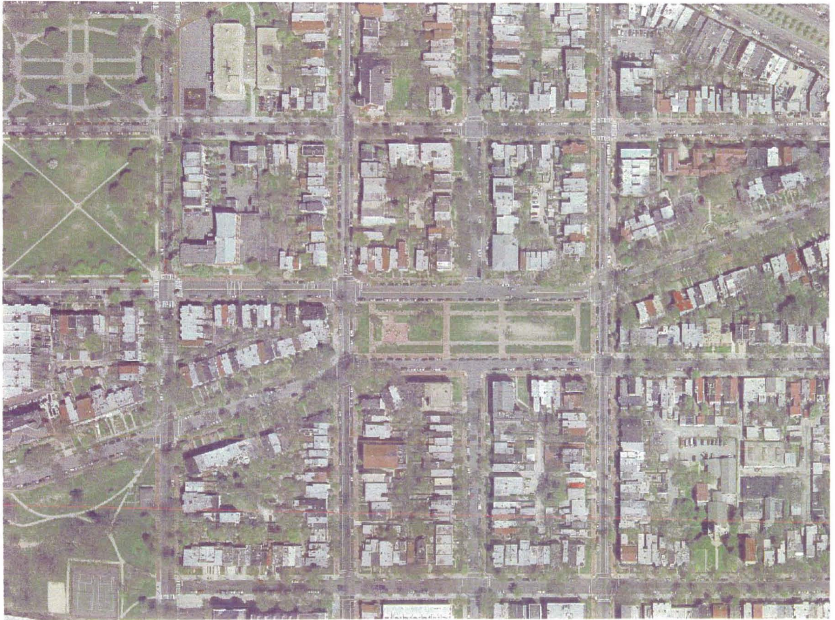
Marion Park (E Street between 4 th and 6 th Streets, SE, including Reservation 18)
