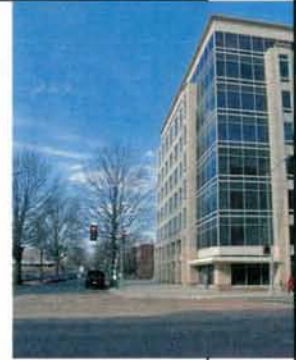
Looking north from the intersection of M Street, SE and 3rd Street, SE 300 M Street office building
