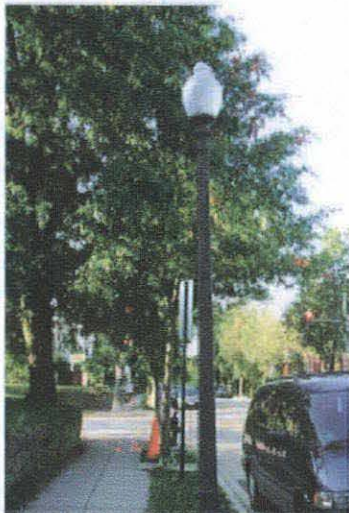
WASHINGTON GLOBE STREETLIGHT
