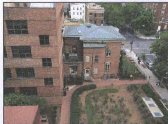
5. VIEW FROM CORCORAN HALL ROOFTOP, LOOKING SOUTH
