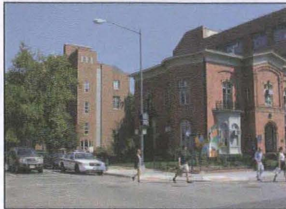
1. VIEW OF SITE, LOOKING NORTHEAST
