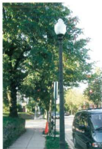
WASHINGTON GLOBE STREETLIGHT
