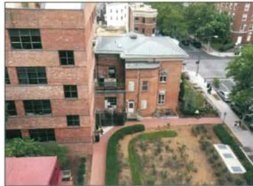
5. VIEW FROM CORCORAN HALL ROOFTOP, LOOKING SOUTH
