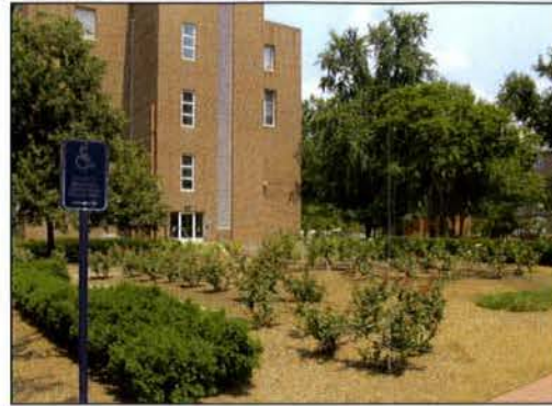
2. VIEW OF SITE, LOOKING NORTHEAST
