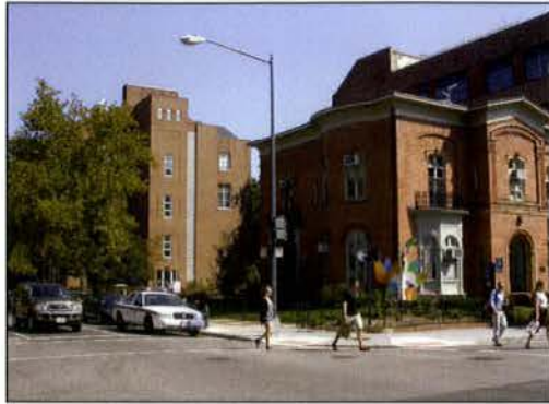
1. VIEW OF SITE, LOOKING NORTHEAST
