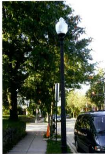
WASHINGTON GLOBE STREETLIGHT
