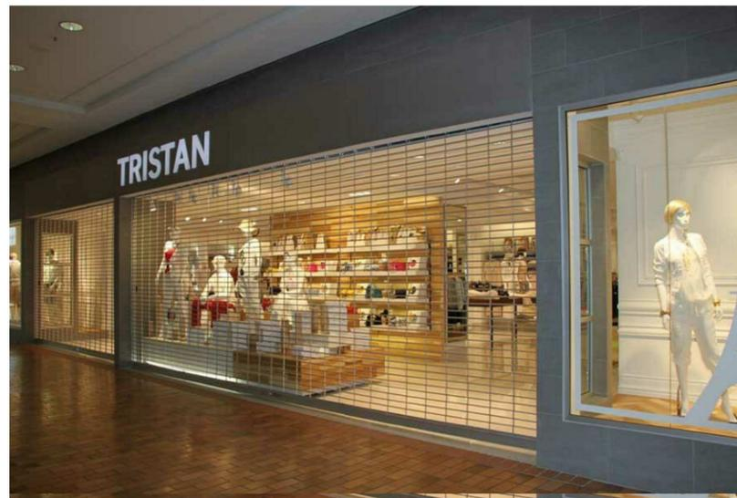
① Security Gate - When open, gate will be full concealed within the architectural housing spanning the opening.
